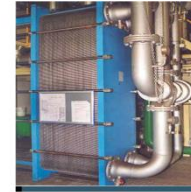
Process Water Cooling at Masterfoods
